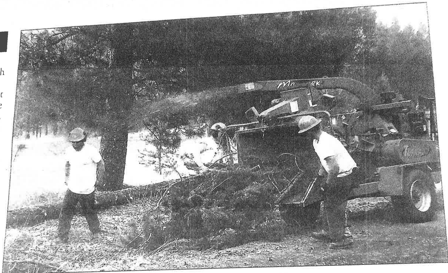
Ladder fuels are often chipped on site and blown onto commons.
