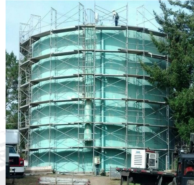
Reservoir Tank Recoating
