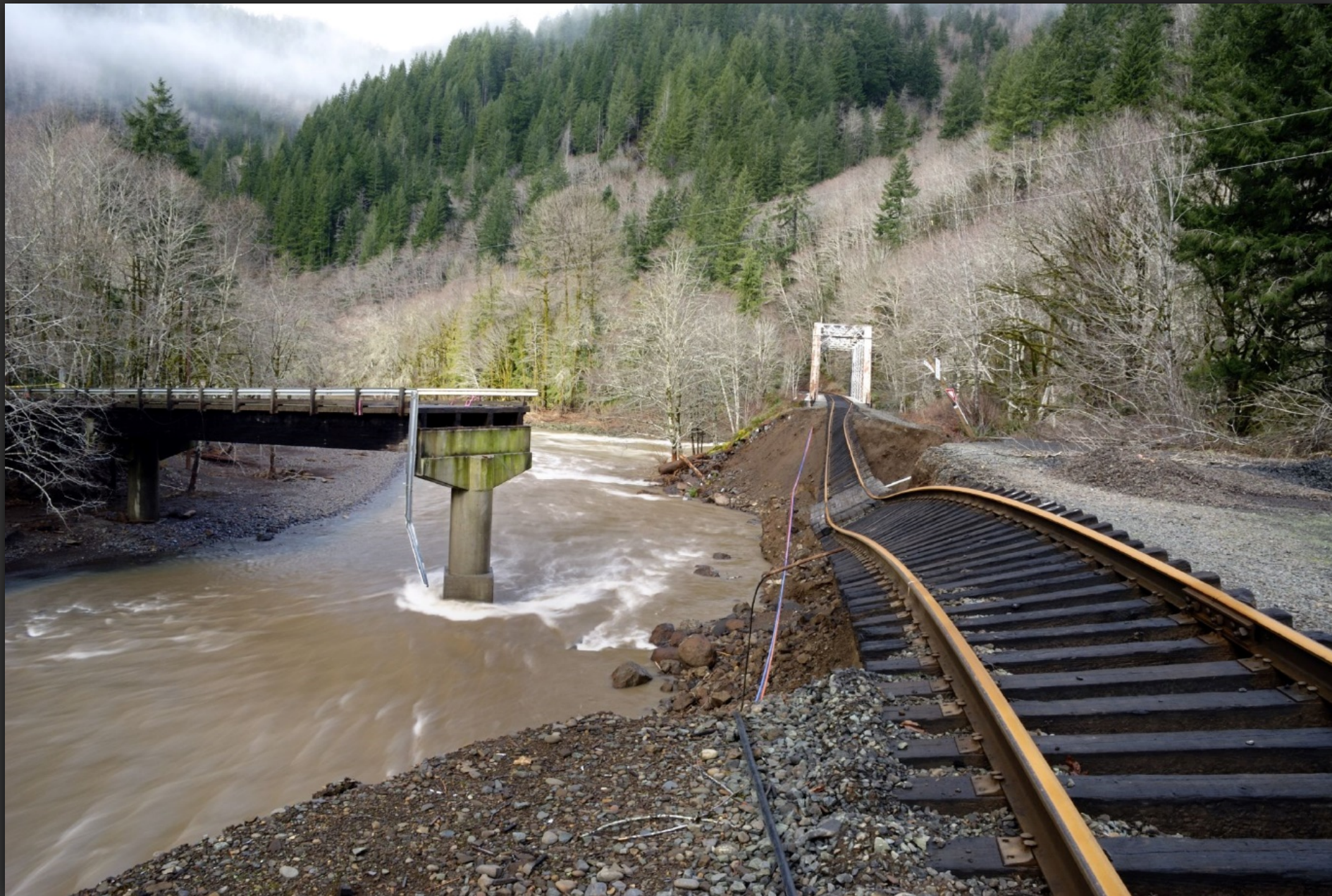
Figure 2: Damage to the Port of Tillamook Bay railroad from channel migration of the Salmonberry River (Courtesy Chris Updegrave, 2/9/2008, https://www.flickr.com/photos/cupdegrave/2253462031/in/photostream/ )
