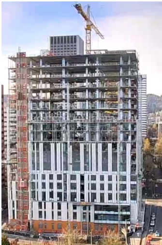
Progress on Multnomah County Circuit Court Courthouse – Dec. 2018
