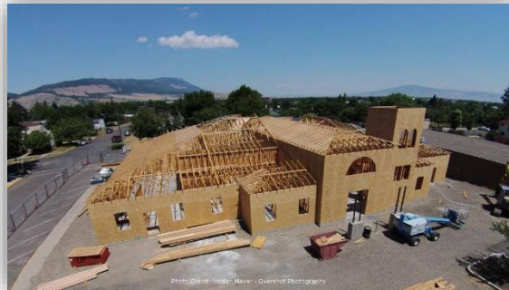
Union County Courthouse construction
