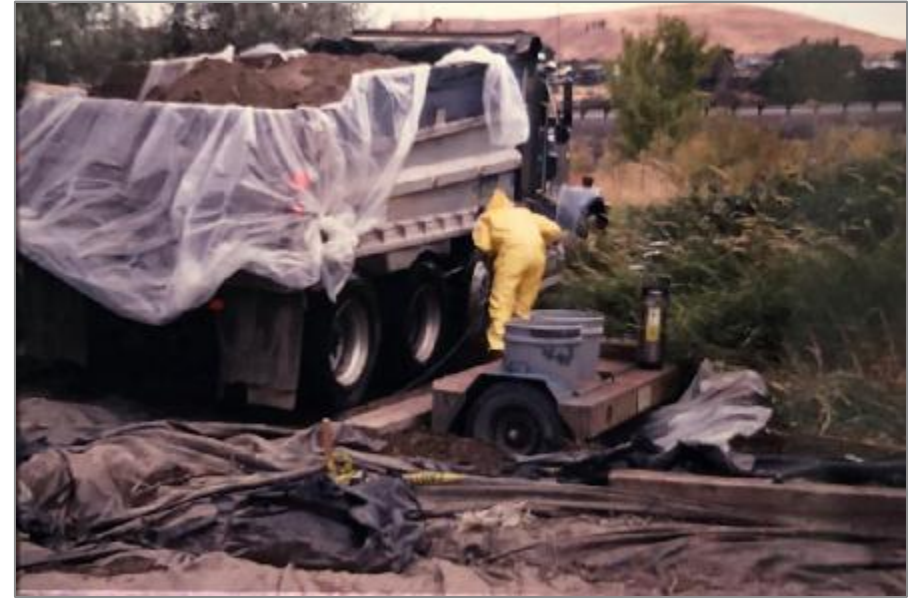
Workers in 1992 removed tons of soil contaminated by the rail tie plant at what is now the city's Riverfront Park.
