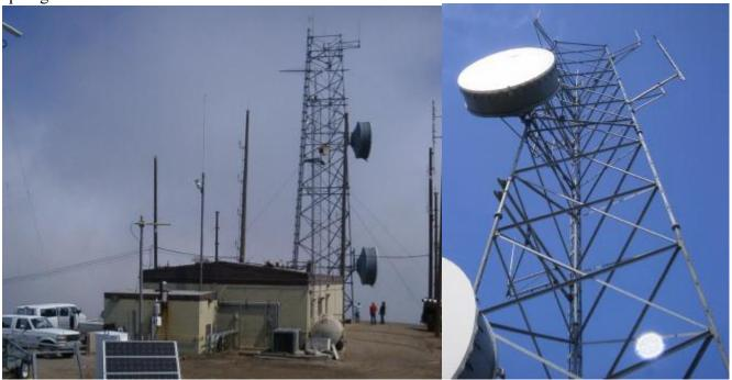
The FCC imposed limit for the license-exempt 5.8GHz band is 53dBm EIRP. The antenna has an about 40dBi gain, and the radio can be software-configured to match the 53dBm limit, taking antenna gain and connector/cable loss estimates into account.
