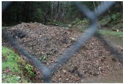
Behind a fence, a recently cleared pile of rock, dirt and twigs sits on the banks of Jetty Creek near the surface water intake for the drinking water plant in Rockaway Beach on Oregon's coast. Coastal storms dumped much of this into the creek. Water quality experts say such storms make coastal communities vulnerable to source water contamination, which they expect to worsen because of climate change.
