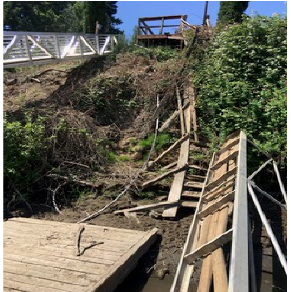
AFTER the High Energy Pounding (2015 – New Ramp on Left)
