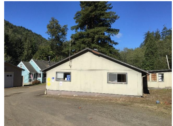
Trask Hatchery Hatch House Replacement
