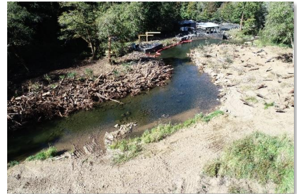
OHRC Bank Repairs
