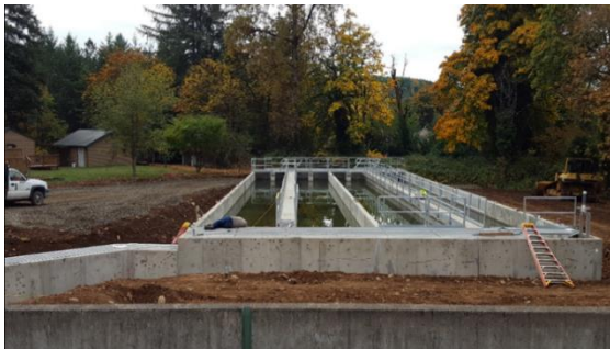
New raceways at Roaring River Hatchery
