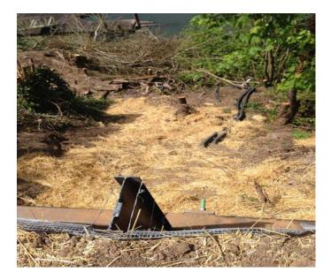
Photo #2 (center of property): Crack in riverbank soil caused the top of the "middle" portion of our riverbank to slide. We installed the first portion of our lower retaining walls at this time. Cost approx. \$14k. February 2016.
