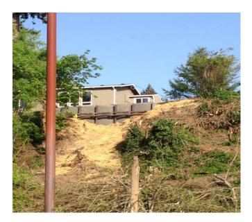
Even with taking our broken pipe and heavy rain into consideration, it seems obvious to us (Photo #3) was augmented by the undercutting of the bank by high energy waves. All retaining wall work was done by PLi Systems, Inc.
