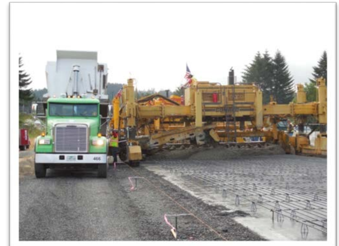
Concrete paving on I-5 near Cottage Grove
