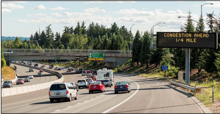
OR 217 Active Traffic Management: Variable Message Signs help convey road conditions to travelers
