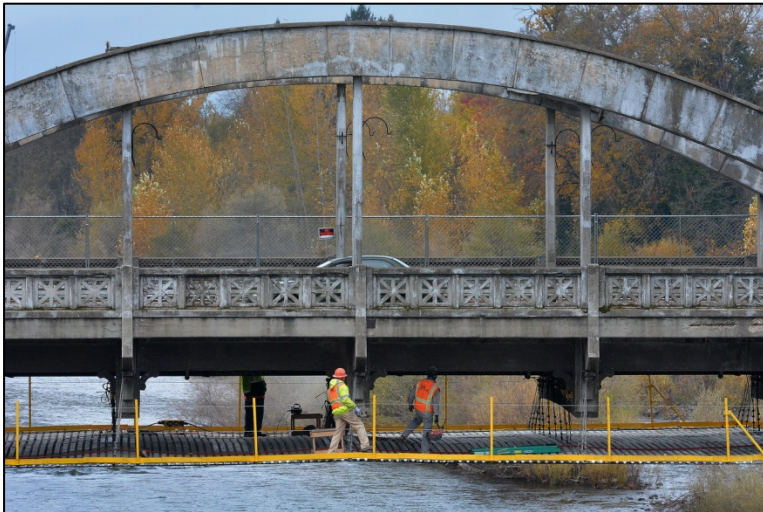
Caveman Bridge (Grants Pass), Josephine County
