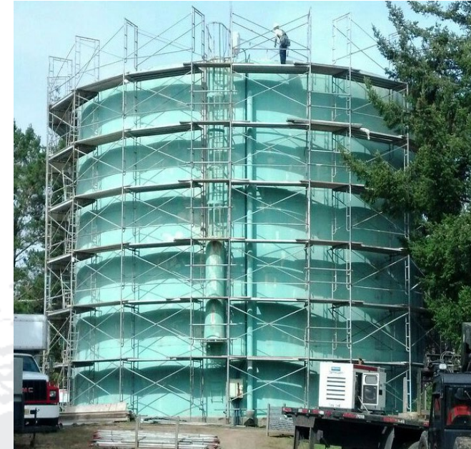
Reservoir Tank Recoating
