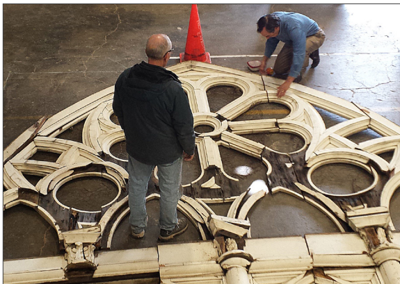
First Congregational Church restoration, Restore Oregon.
