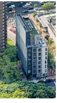
The Carmel Place building is composed of four staggered, 11-foot-wide towers, each corresponding to a column of stacked modules. Bricks in four shades of gray were chosen for the facade.
