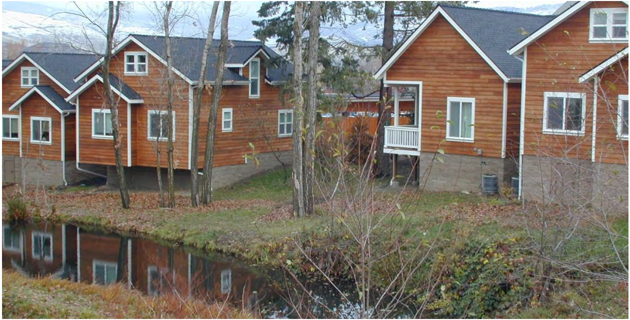
Figure 35. Ashland Creekside Housing.
