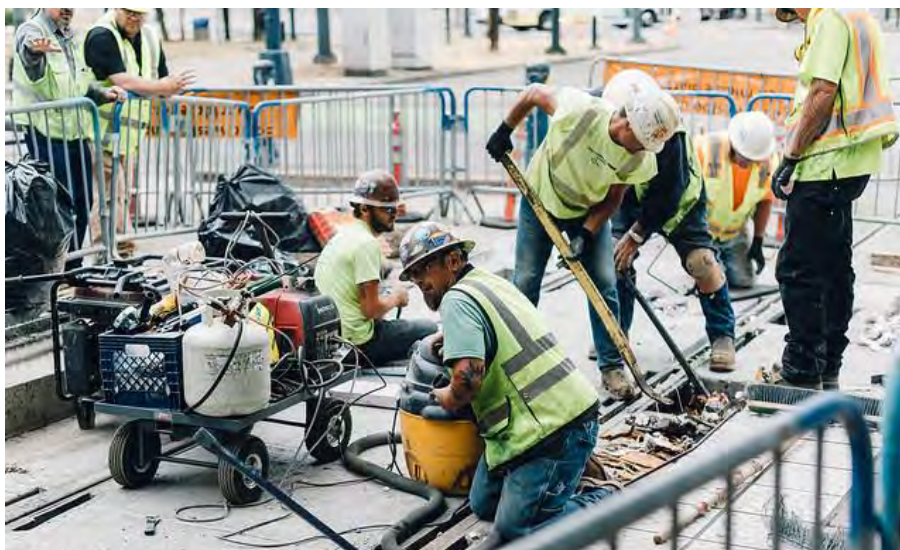
Figure 16. Work on Rose Quarter MAX line, Portland
