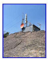
Translator: A broadcast transmitter device which repeats the signal of a radio or television station to an area not covered by the signal of the originating station.
