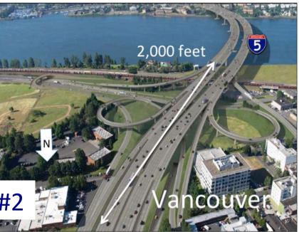
"Columbia River Crossing" bridge design comes down from over 150 feet, and requires almost half-a-mile of elevated concrete viaduct on both bank to connect to current highways
