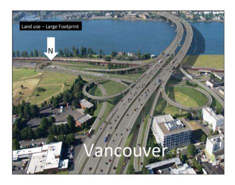
3. An Immersed Tube Tunnel has less land impact than a High Bridge
