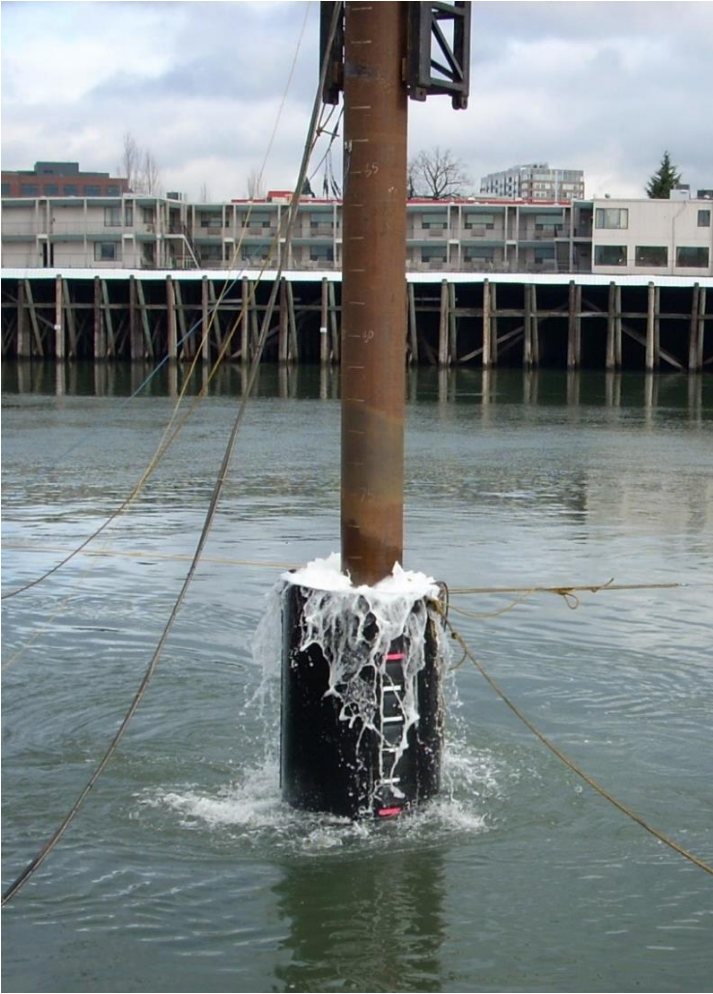
Confined bubble curtain from Test Pile Project
