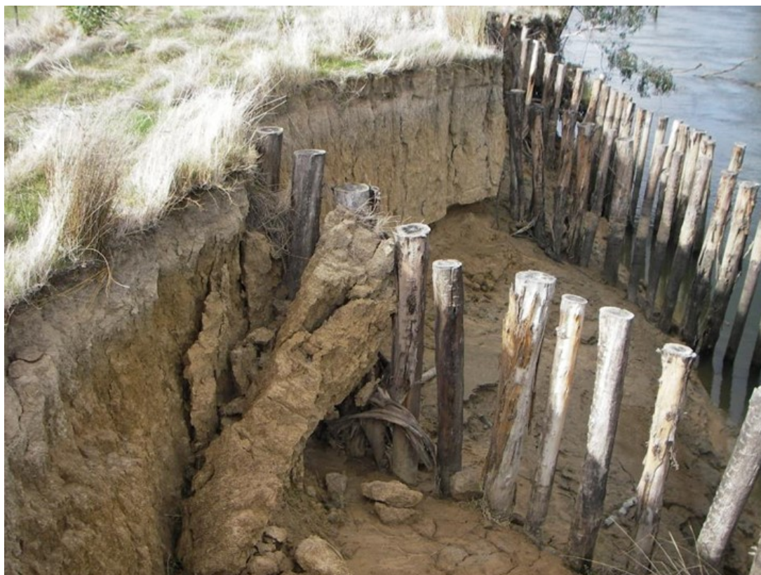
Figure 18: Bank sheering behind pile fields.
