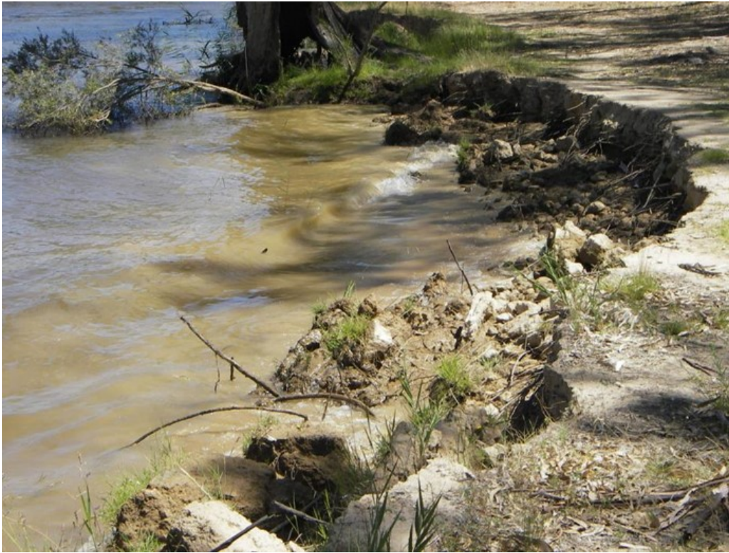
Figure 15: Steep bank erosion with waves breaking.
