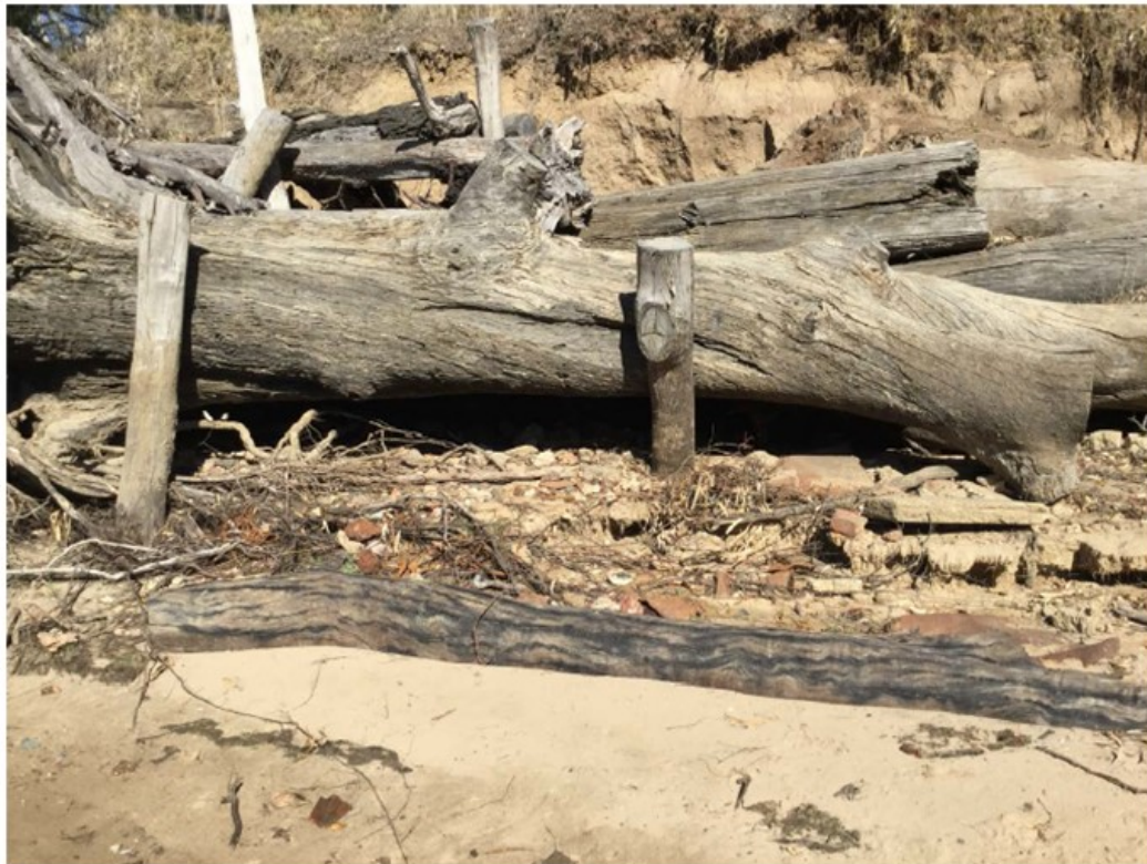
Figure 11: Ball Park log revetment undermined from boat wash.
