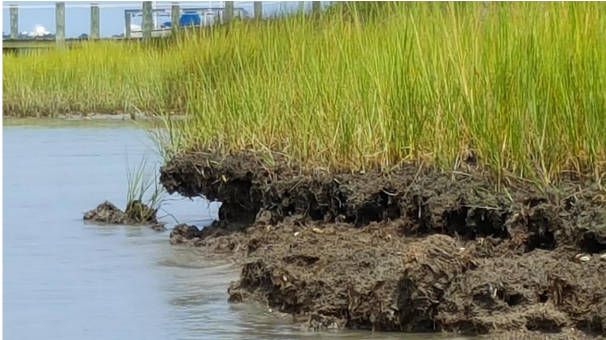
Figure 6. Marsh erosion reportedly induced by boat generated waves on Lynnhaven River, Virginia. Photo by Bill Fleming.
