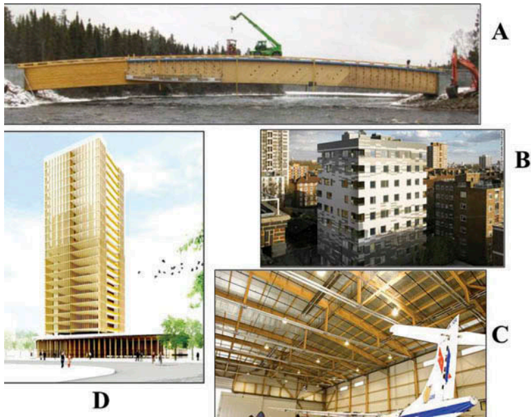
FIGURE 1 Innovative wood construction designs can replace much steel and concrete: (a) high-load wood bridge, Quebec, Canada; (b) Stadthaus—Murray Grove Tower, London, United Kingdom; (c) aircraft hanger in Montreal, Canada; (d) design of 20-story wood building, Vancouver, British Columbia, Canada. ((a) and (c) construction by Nordic Engineered Wood, Chantiers Chibougamau, LLC, Quebec; photo courtesy of Jean-Marc Dubois. (b) designed by Waugh Thistleton Architects, London; photo courtesy of Will Pryce, London. (d) of designed building, MGA, Michael Green Architecture, Brooklyn, New York, and Vancouver, British Columbia.)
