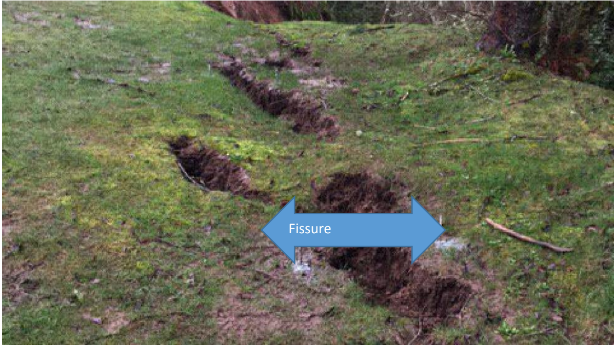
March 2017 Landslide – Mt. Calvary Cemetery, Portland
