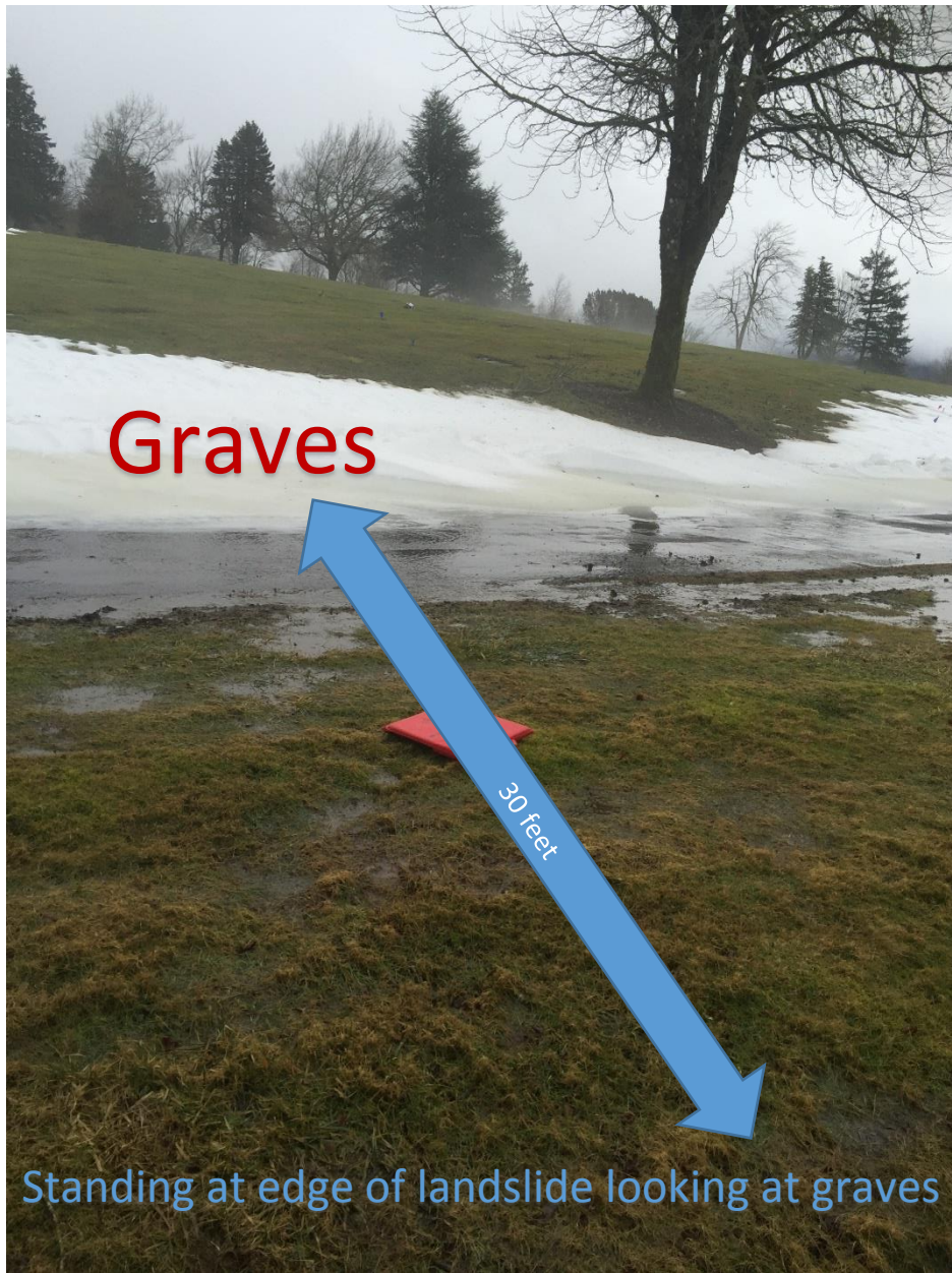
January 2017 Landslide at Skyline Memorial Gardens, Northwest Portland. Over 1,500 yards of earth
