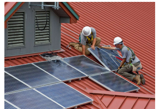
Contractors installing solar panels
