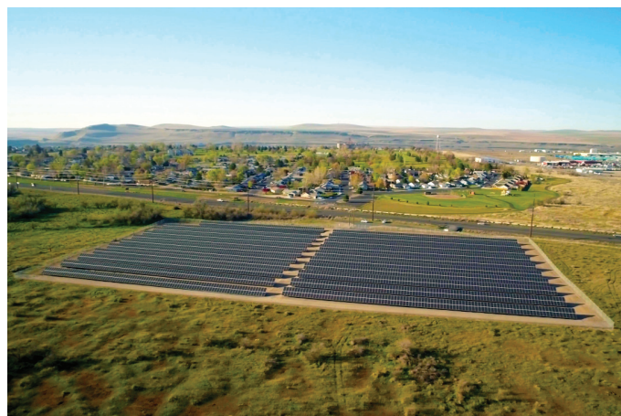
The Umatilla Electric Cooperative constructed a solar energy generating plant on the eastern edge of Umatilla, Oregon.
