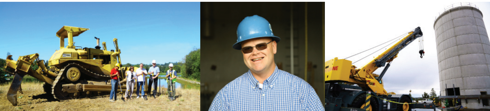
From left to right: the town of Vernonia breaks ground on its wastewater system improvement project; Crooked River Ranch Water Company Manager Frank Day visits the elevated water storage tank construction site; the pedestal for the Crooked River Ranch water tank during construction.
