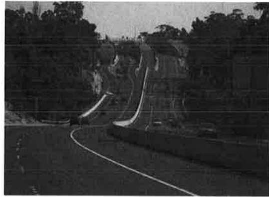
M2 Motorway, Australia
