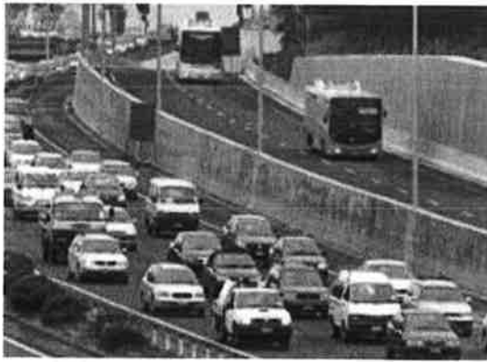
SH1 Northern Busway, Auckland 18
