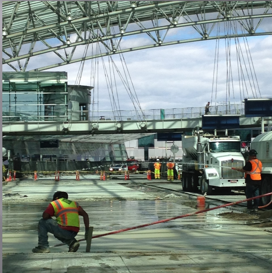
PDX Airport Upper Deck Repair by Volumetric Mixer
