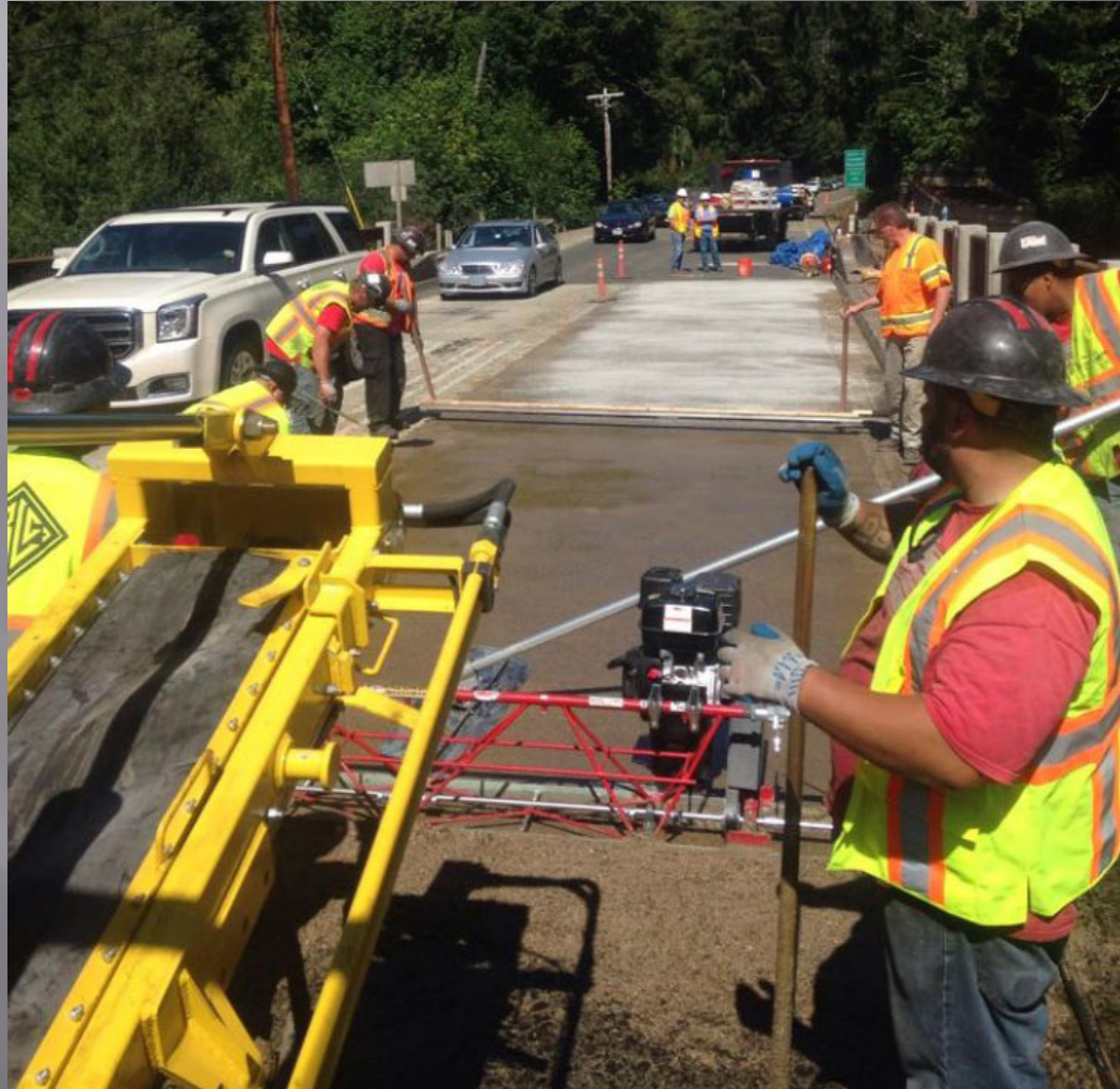
Pouring Necanicum bridge deck overlay on Hwy 26 by Volumetric Mixer
