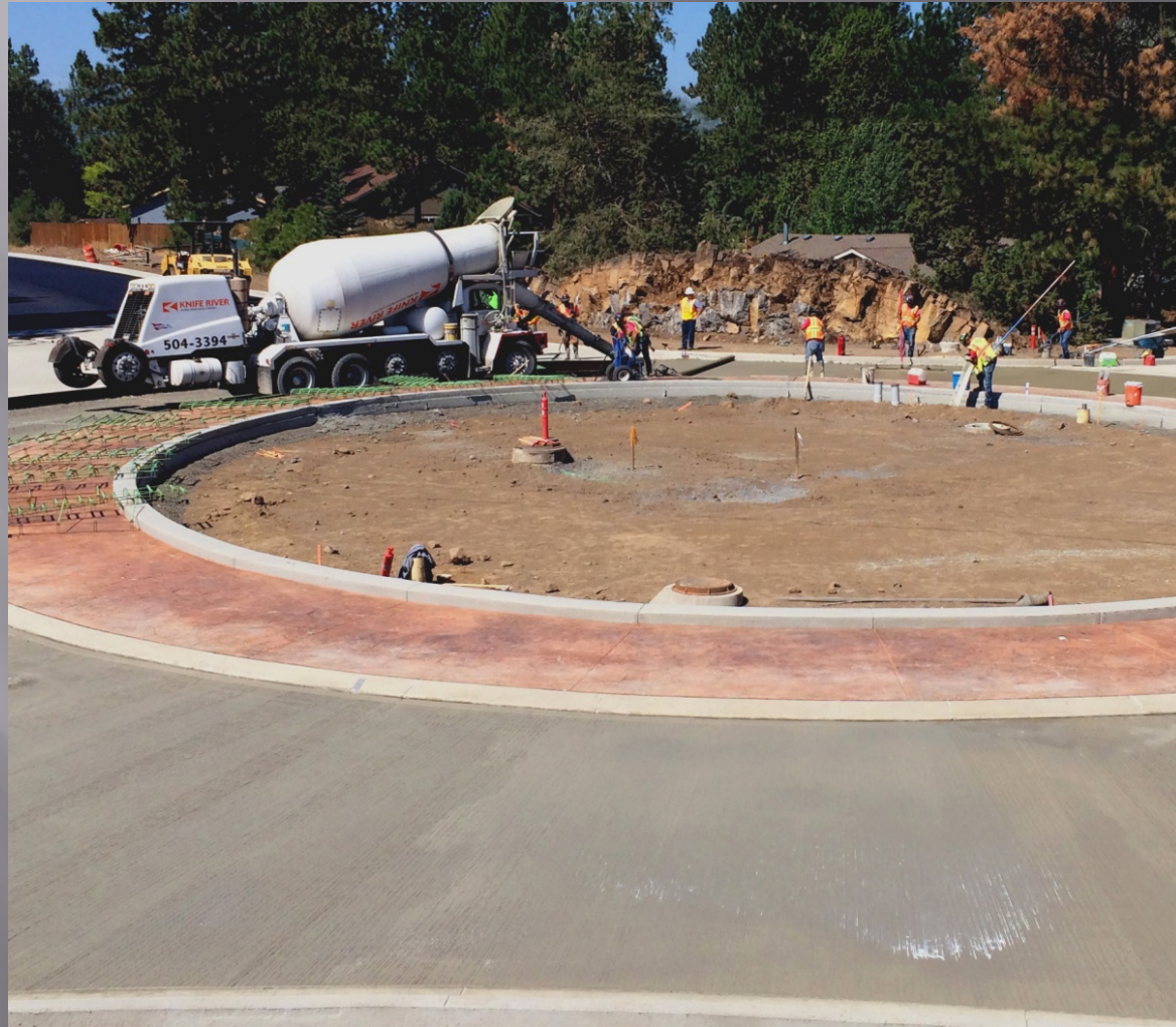
Roundabout Intersection Pour by Transit Mixer
