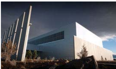
Facebook’s data center in Prineville.
