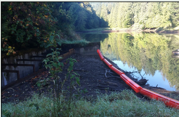
Silt and debris builds up, creating "Sand Island." Water is then too low to spill over the dam.
