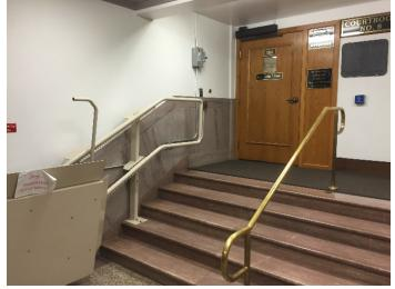
Stairs up to courtroom and non-functioning lift due to inadequate existing wall bearing capacity
