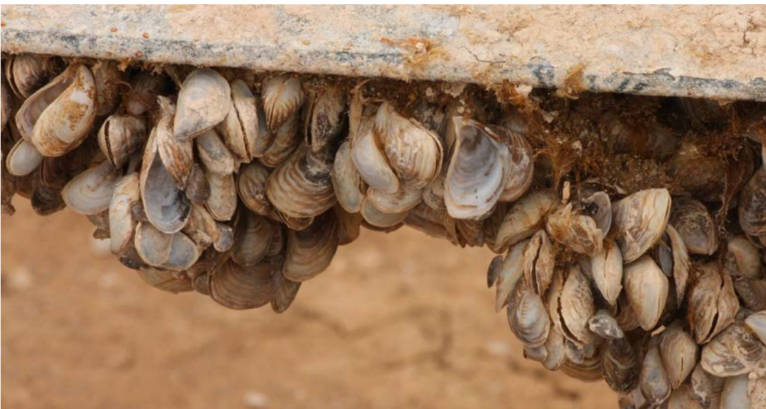
Figure 12: A magnified view of Quagga mussels on a marina support structure now above the waterline. Credit ©: J. N. Stuart via Flickr.
