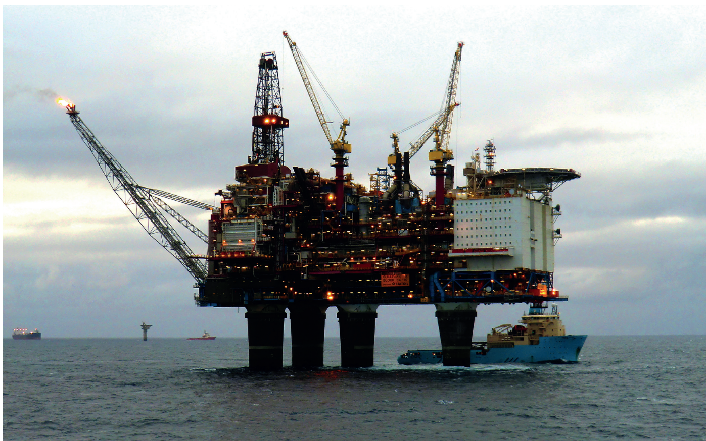
Gullfaks Alpha, the oldest of three platforms operated by Statoil in the Gullfaks oil and gas field.
