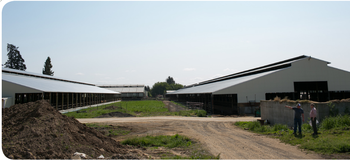
Waste from Forest Glen Oaks' dairy cows is used to produce biogas and generate renewable electricity at the Dayton farm.
