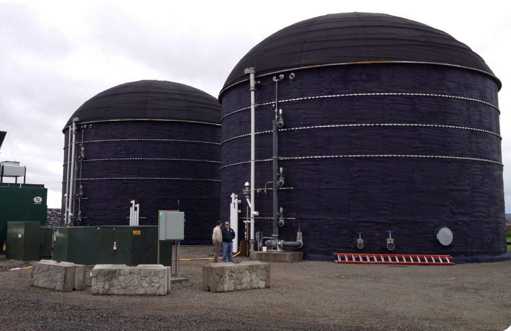
Project owner Revolution Energy Solutions uses digester tanks like these to transform 50,000 gallons of cow manure per day into renewable energy.
