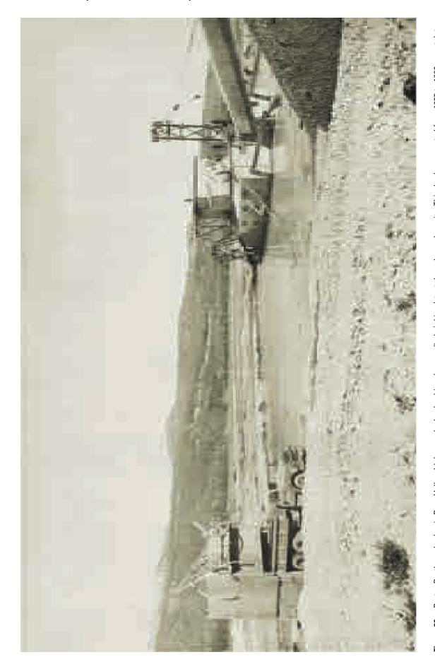
of photograph is unknown. Monazite was produced as a byproduct from these placer deposits. (Photograph from Savage (1961, fig. 13); used with permission of Idaho Geological Survey.) Figure 20. Porter Brothers dredge in Bear Valley, Idaho, worked columbium (now called niobium)-tantalum placer deposits. This dredge operated from 1955 to 1960; exact date
