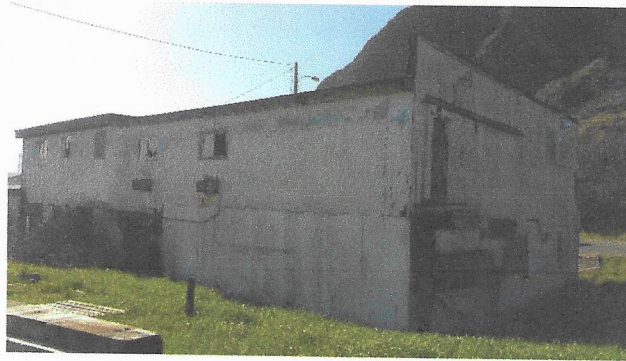
Existing Structure Exterior
