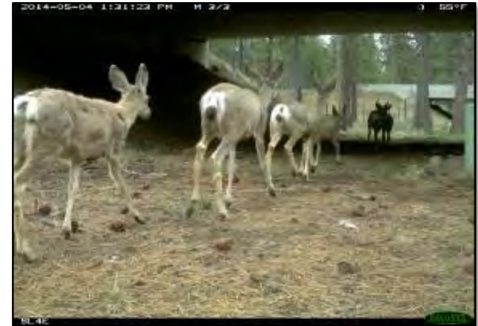
Wildlife underpass on Highway 97
