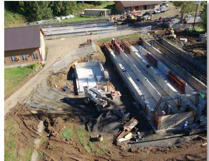
Cedar Creek Hatchery: Partially constructed ponds as of October 2016.
