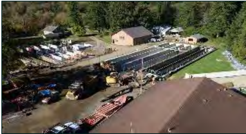
New raceways at Cedar Creek hatchery
