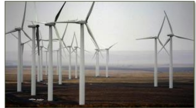
Wind Farm near Arlington
