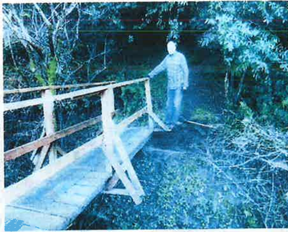
One of the completed bridges.
