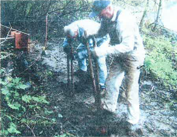
Digging holes for bench.
