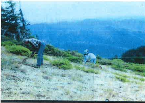
Trail crew building east spur trail to Brandy Peak
