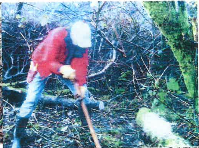
Kathie digging tread.
