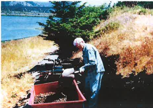
Cliff Burges loading gravel
