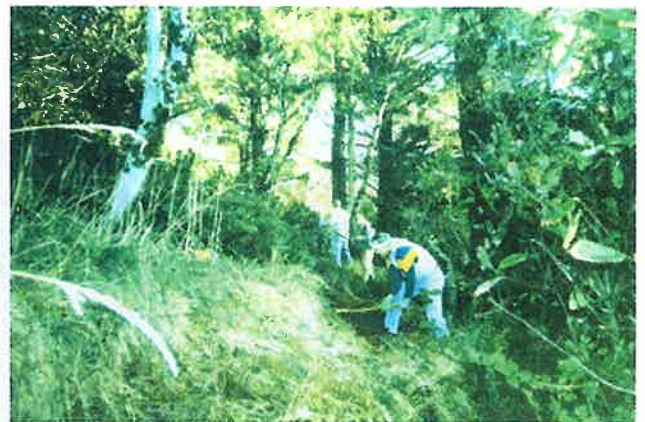
Digging a new trail at Otter Point to replace Section taken out by slide.
