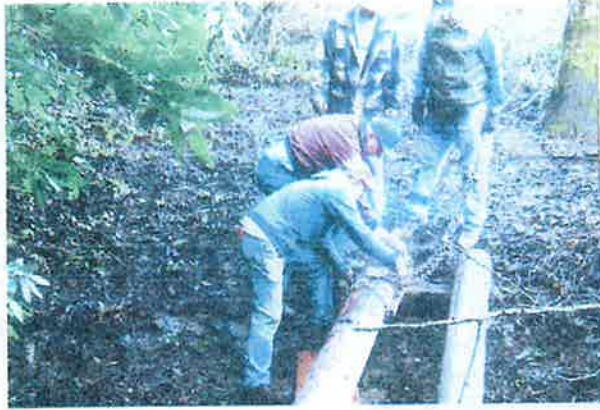
Placing power poles for bridge stringers. Photo by Al Collinet
