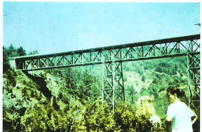
A side trail goes to this Thomas Creek Bridge view.
