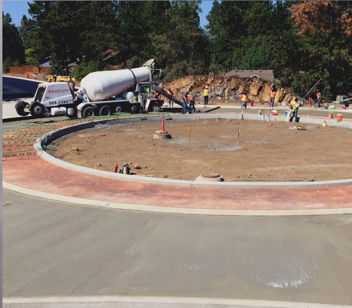
Roundabout Intersection Pour by Transit Mixer
