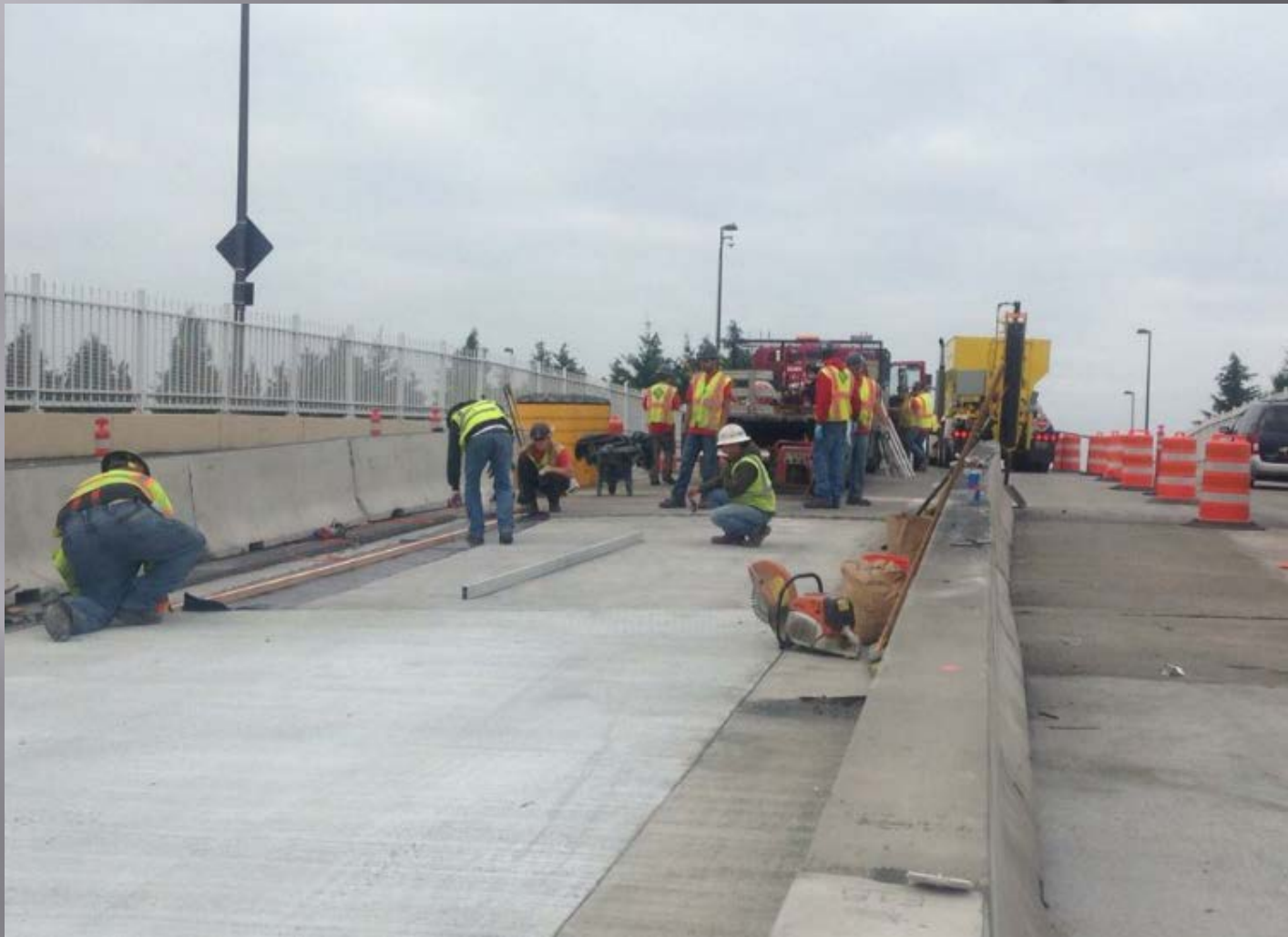
Interstate 5 Overpass at Woodburn: Project poured by Volumetric Mixer
