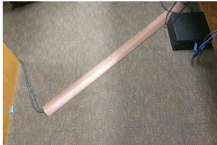
Cables at litigation well in courtroom
