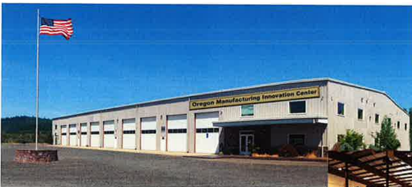
Figure B: OMIC R&D Facility in Scappoose, OR. Representative signage added.
