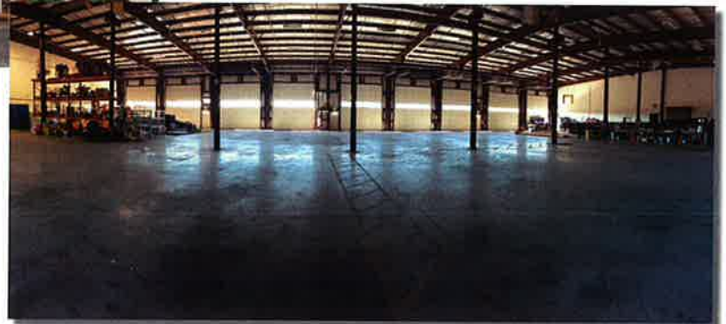
Figure C: OMIC R&D High Bay Interior View
