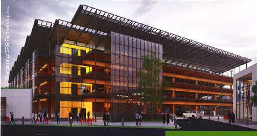
Pictured from top to bottom: Richard Woodcock Education Center, Glenwood Parking Structure and Carbon12.
