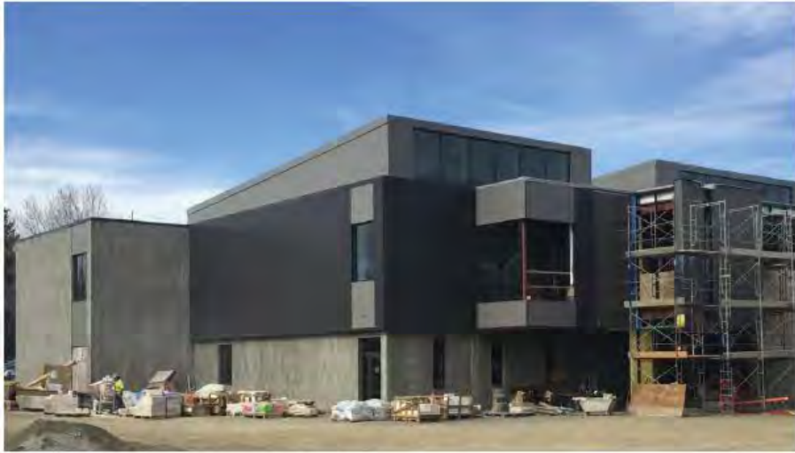
Exterior of the new Jefferson County Courthouse - early phase of construction.
