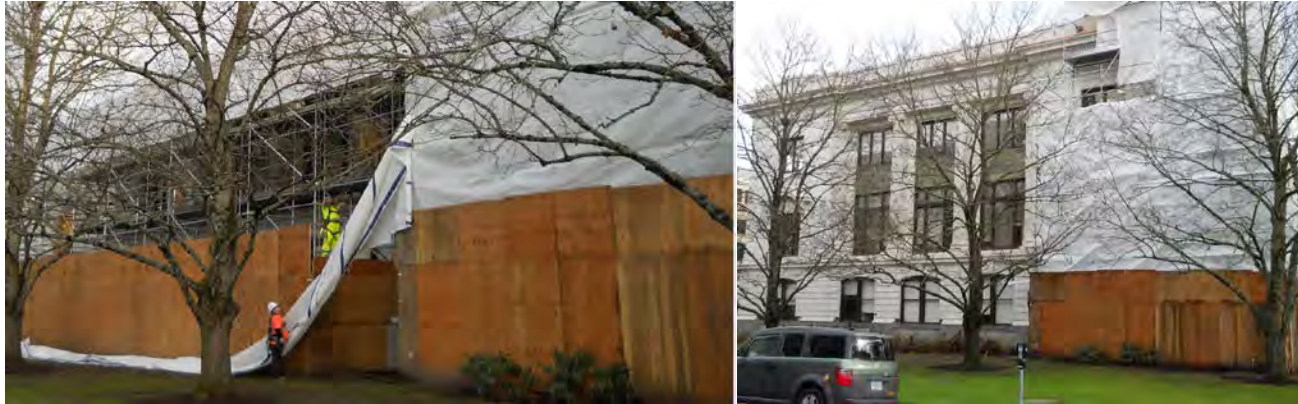
Scaffolding and protective cover for work
