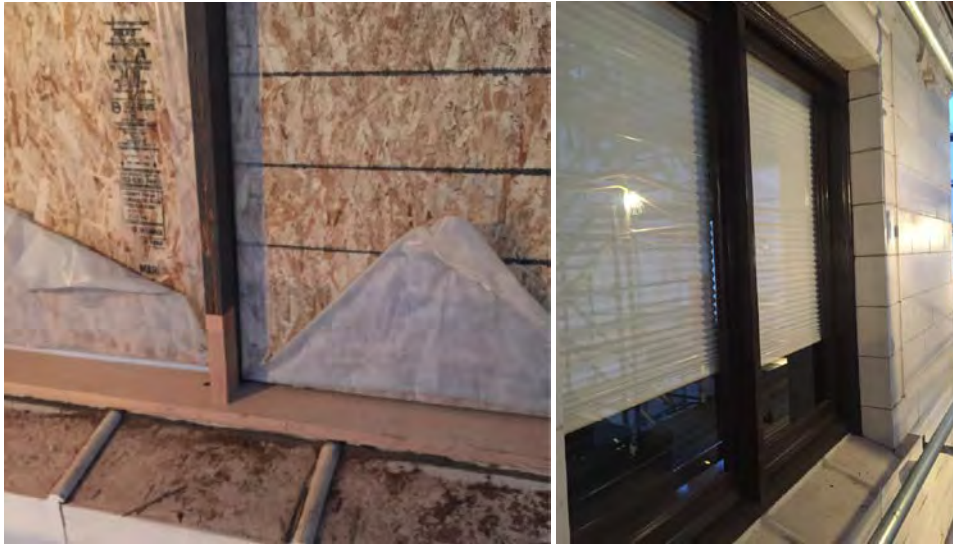
Windows, framing repair and replacement
