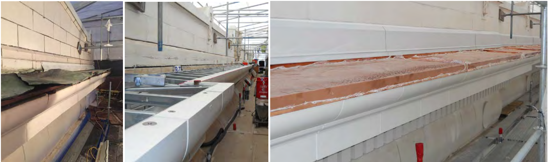
Work on cornices, structural supports, tile, flashing
