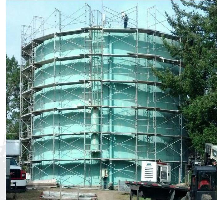
Reservoir Tank Recoating
