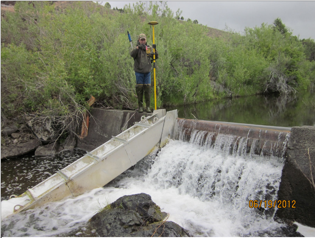
Irrigation diversion depicted above was replaced with a Low Head Diversion and an Engineered Riffle providing natural fish passage depicted to the right.
