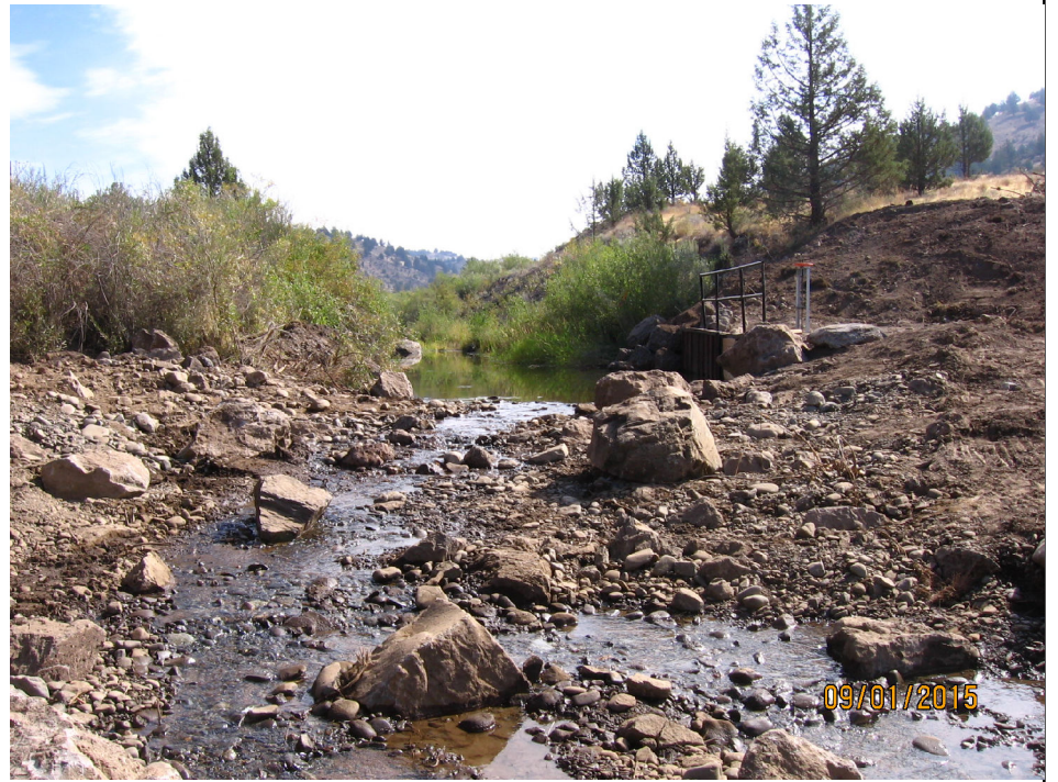
Irrigation diversion depicted above was replaced with a Low Head Diversion and an Engineered Riffle providing natural fish passage depicted to the right.
