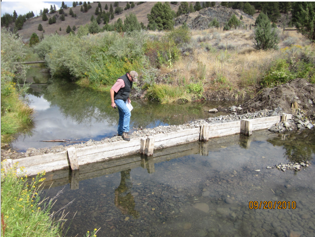
Irrigation diversion depicted above was replaced with a Low Head Diversion and an Engineered Riffle providing natural fish passage depicted to the right.
