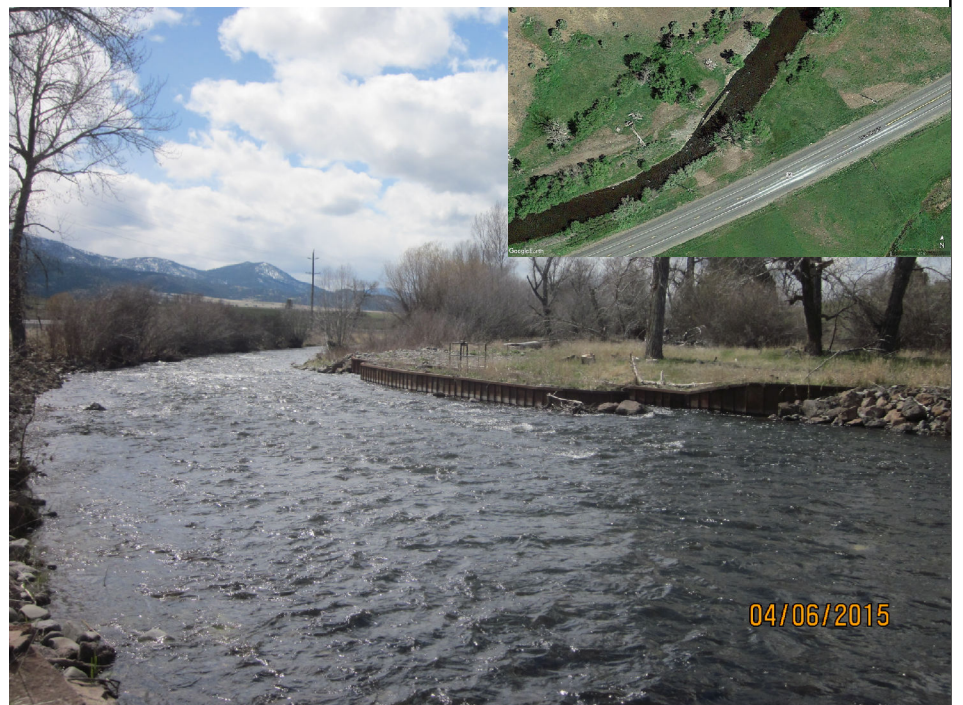
Irrigation diversion depicted above was replaced with a Low Head Diversion and an Engineered Riffle providing natural fish passage depicted to the right.
