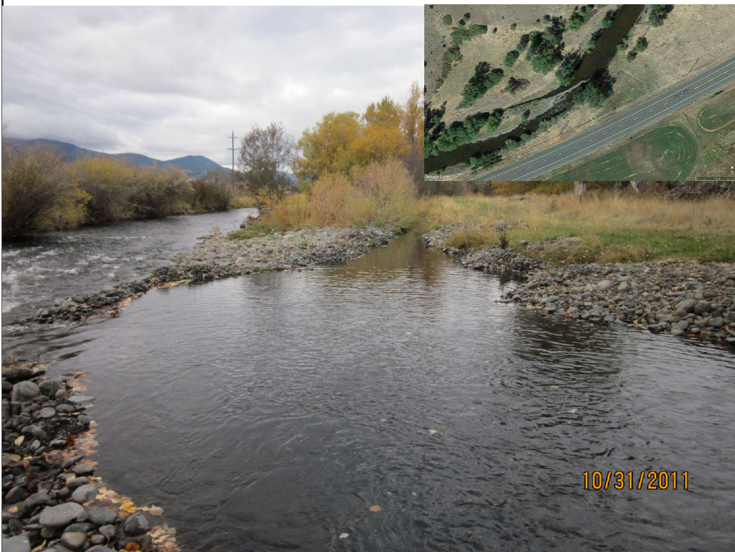
Irrigation diversion depicted above was replaced with a Low Head Diversion and an Engineered Riffle providing natural fish passage depicted to the right.
