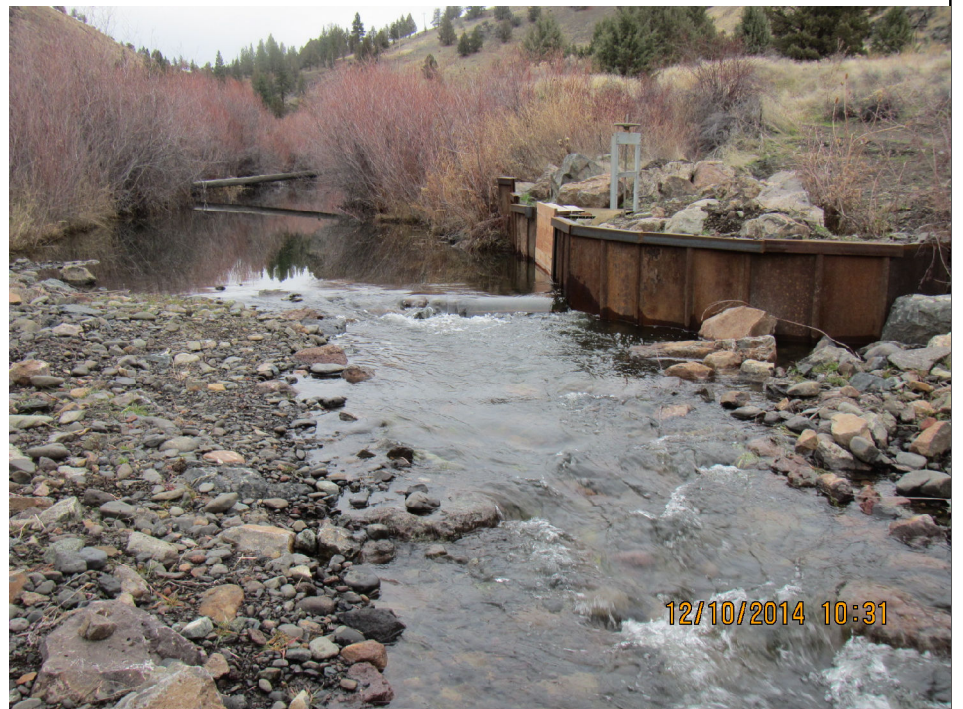
Irrigation diversion depicted above was replaced with a Low Head Diversion and an Engineered Riffle providing natural fish passage depicted to the right.
