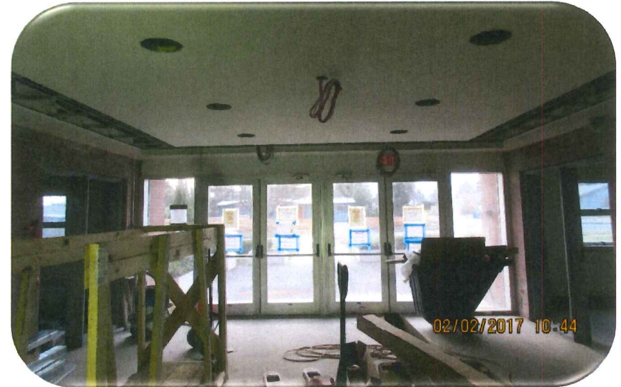
Maison Armory (North Portland) Project completion: April 2017
