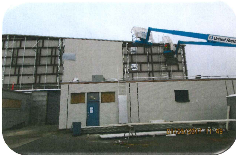
Medford Armory Service Life Extension Plan Project completion: April 2017
