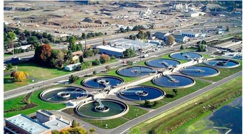
Wastewater Treatment Facility, Eugene, OR
